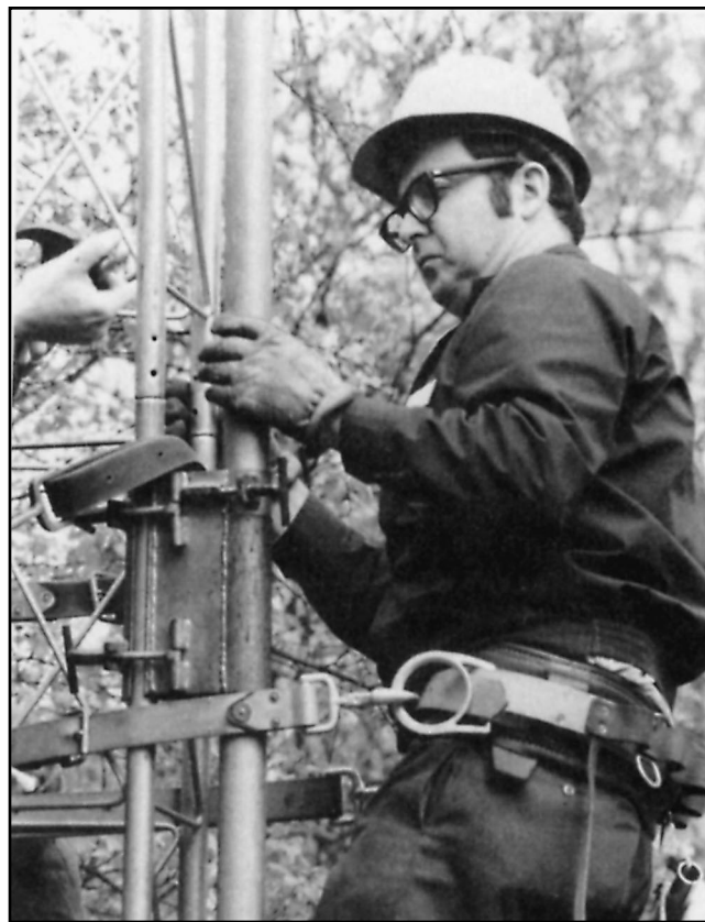
Fig 1—Bill Lowry, W1VV, uses a good quality safety belt, a requirement for working on a tower. The belt should contain large steel loops for the snap straps. Leather loops at the rear of the belt are handy for holding tools. (photo by K1WA)
